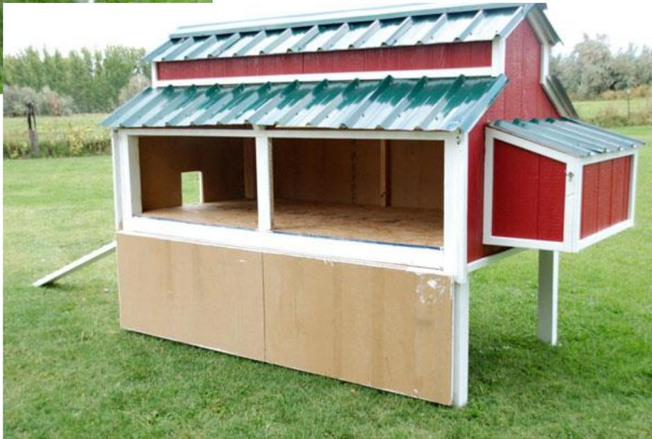
10. You'll also need a ramp for the chickens to get into the coop. Cut a hole (about 10" x 10") in the back of the coop, 3 3/4" from the bottom.
