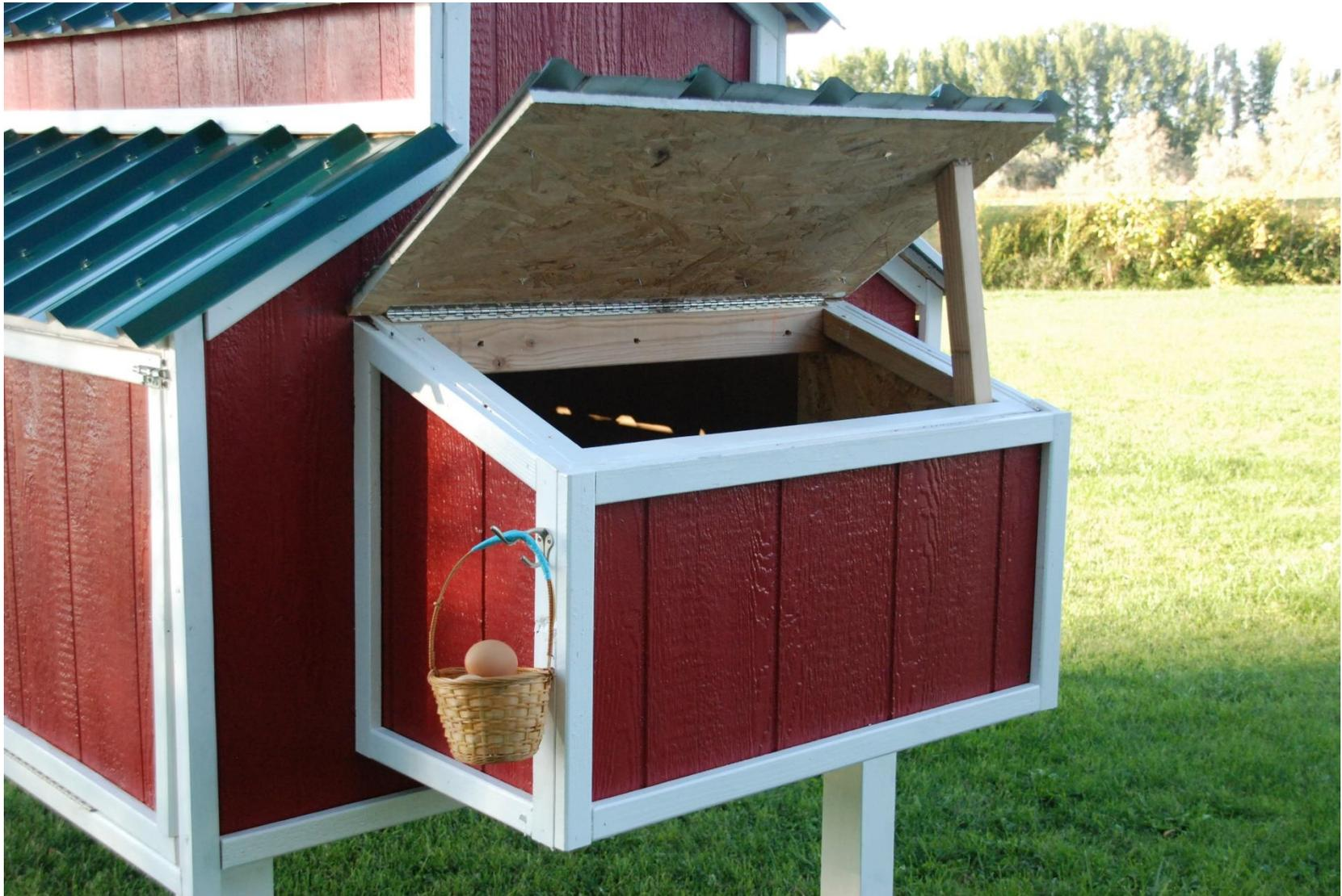
9. Once our nesting box is complete, we can attach the side that folds down. You might need a helper to hold the side up in place while you screw the piano hinge on. Screw a couple of screws in, then hinge it up and make sure it's straight before you finish screwing in all the rest of the screws.
